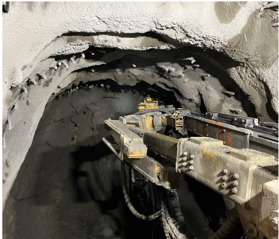
Shotcrete and Spilings at Crosscut Heading
