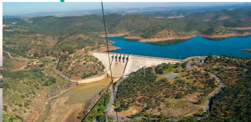
Andevalo Hydroelectric/Water Dam
