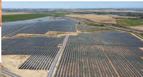
Paymogo Solar Power Plant
