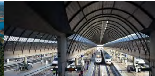
Huelva-Sevilla-Madrid Rail Station
