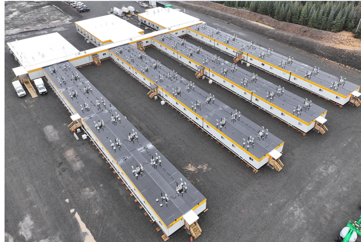
CAMP 11 WORK AREA
